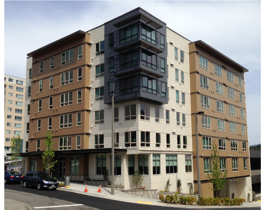
August Wilson Place 57 workforce apartments
